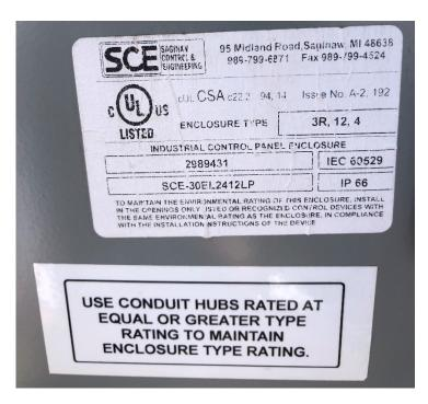
Figure B.4 - Control Panel Enclosure Information
