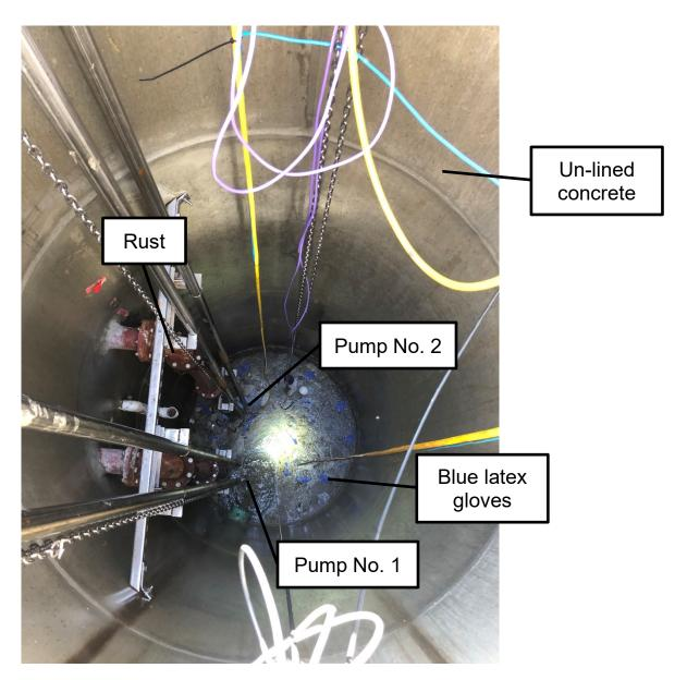
Figure 3 - Inside RVSLS Wet Well
