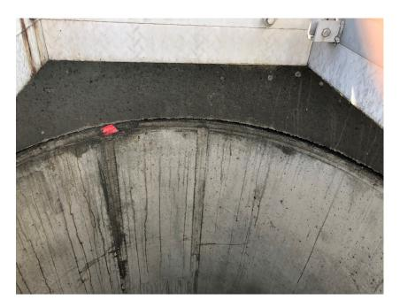
Figure 5 – Possible Signs Of Infiltration Through The Concrete Joints
